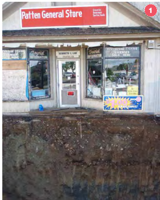
#1. Phase 1 soil excavation at the "door yard" of Patten General store.
