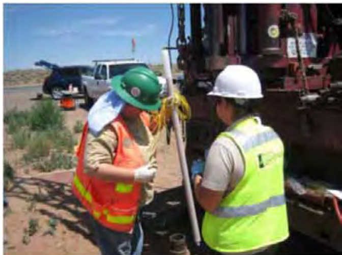
Remediation work at Navajo Nation, Arizona.
