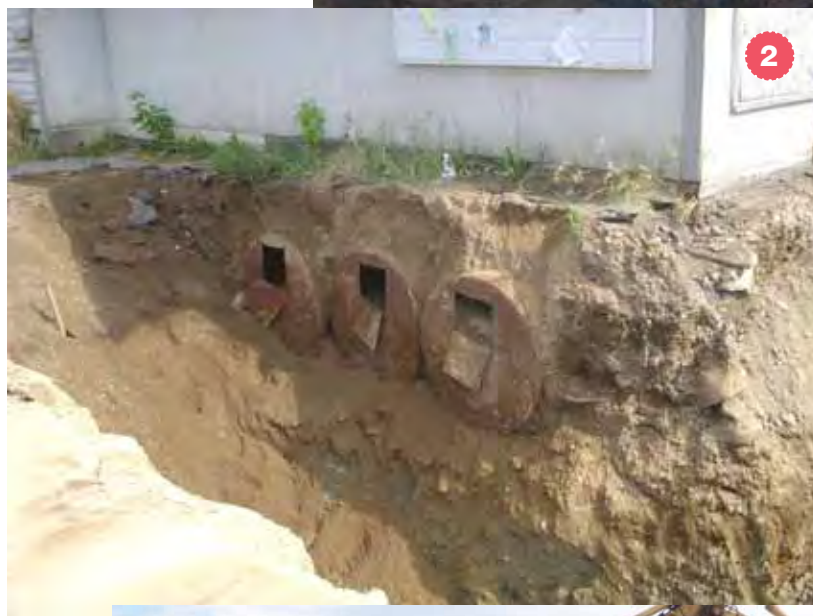
#3. The store is demolished and Phase 2 soil removal begins.
